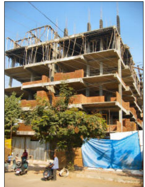
A construction site in India
